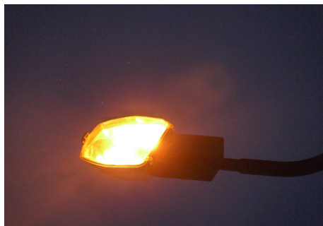
Sodium vapor lamp is more safe than the mercury vapor lamp
